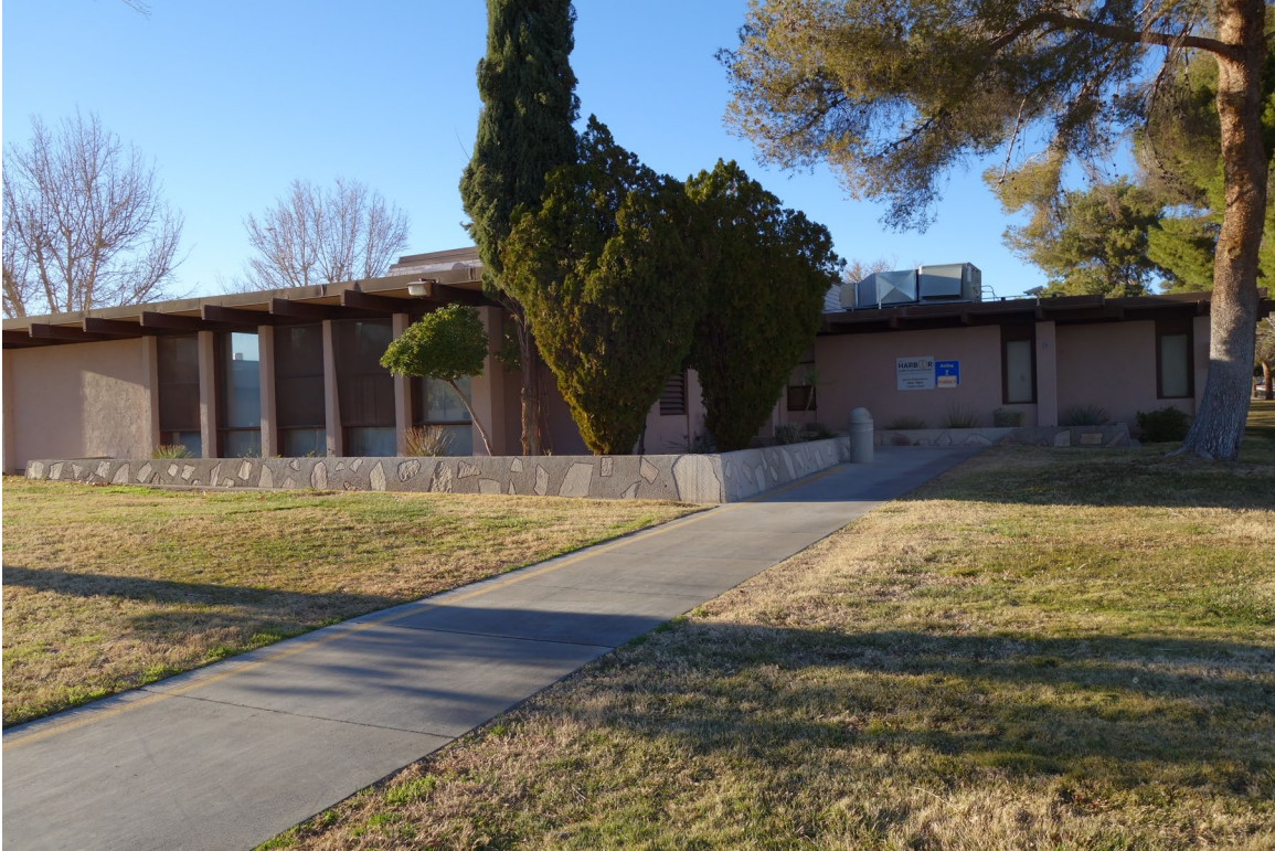
#2 Pharmacy / Laboratory Building – FCA Building #0243 Description: Window Replacement Needed.
