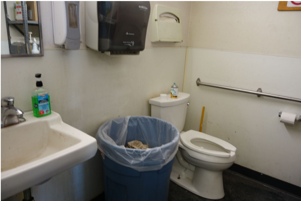
#6 Storage / Shop – FCA Building #1954 Description: ADA Restroom Upgrade Needed.
