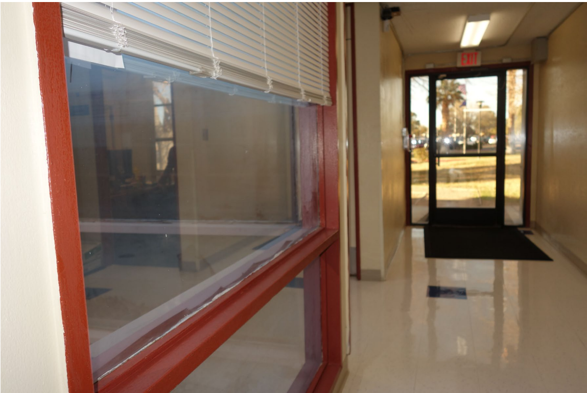
#1 Administration / Outpatient Services – FCA Building #1949 Description: Single Pane Windows Replacement Needed.
