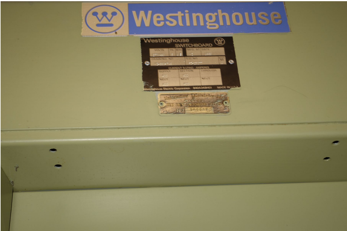
#2 Pharmacy / Laboratory Building – FCA Building #0243 Description: Electrical Upgrade Needed.
