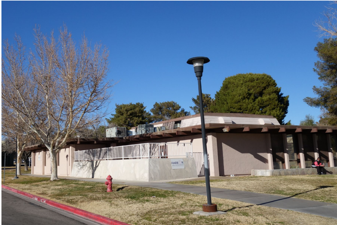
#2 Pharmacy / Laboratory Building – FCA Building #0243 Description: Exterior of the Building.
