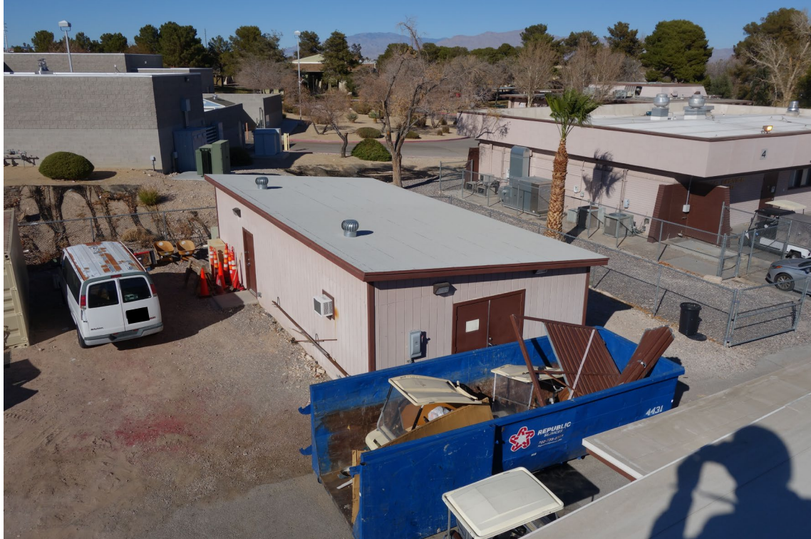
#6A Storage Building – FCA Building #0360 Description: Exterior of the Building.
