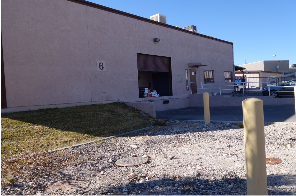
#6 Storage / Shop – FCA Building #1954 Description: Exterior of the Building.
