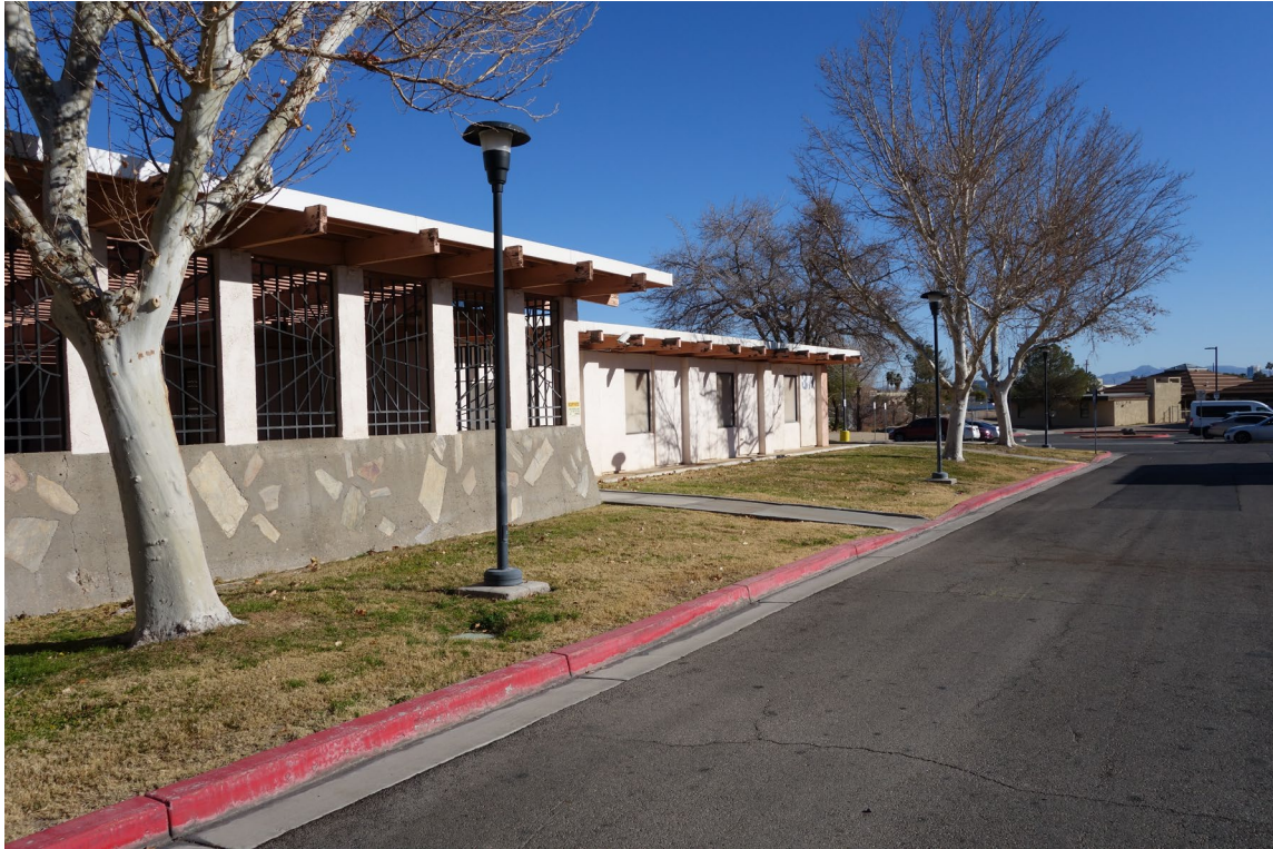
#3A Crisis Observation Unit – FCA Building #1951 Description: Exterior of the Building.
