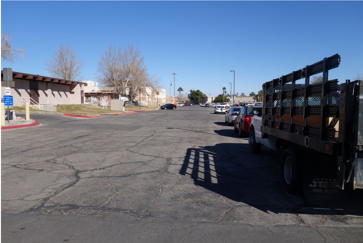
Southern Nevada Adult Mental Health Services Site – FCA Site #9992 Description: Transverse Drive Rehabilitation Needed.
