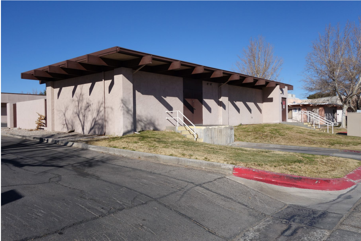
#5 Food Service Center Storage – FCA Building #1953 Description: Exterior of the Building.
