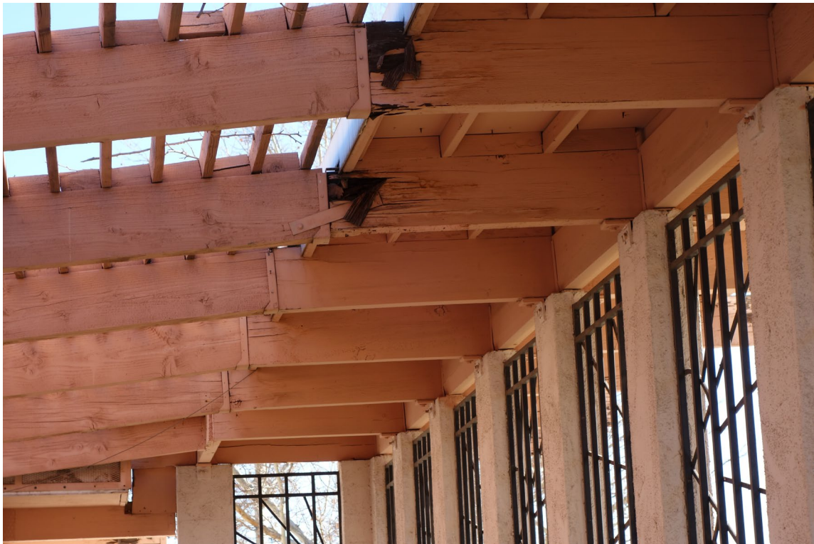
#3A Crisis Observation Unit – FCA Building #1951 Description: Structural Assessment of Shade Canopy Needed.
